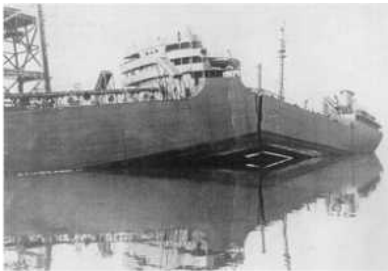
FIG. 19 EXAMPLE OF BRITTLE FRACTURE IN SHIP STRUCTURES
